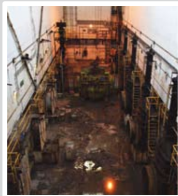
The clearance of the Hinkley Point A Cooling Water Pumphouse
