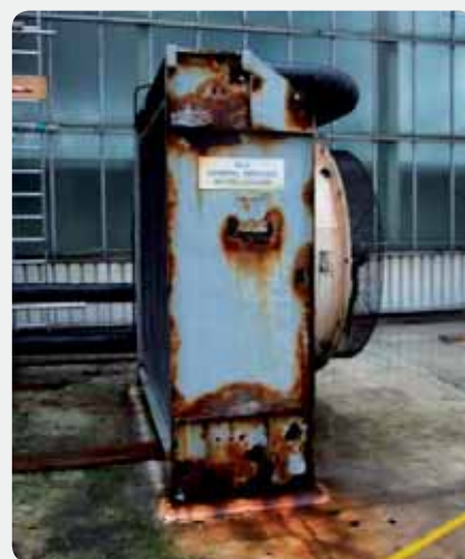
Dungeness plant is exposed to coastal elements
