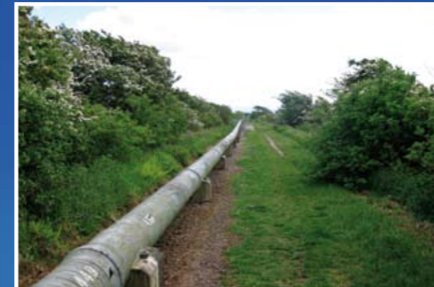
The pipeline which stretches from the Site to the Solway Firth
