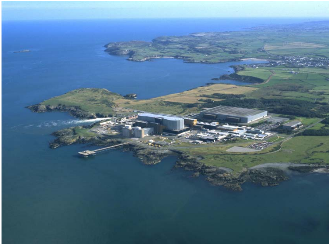
Photograph 1: View of Wylfa Nuclear Power Station and Surrounding Area
