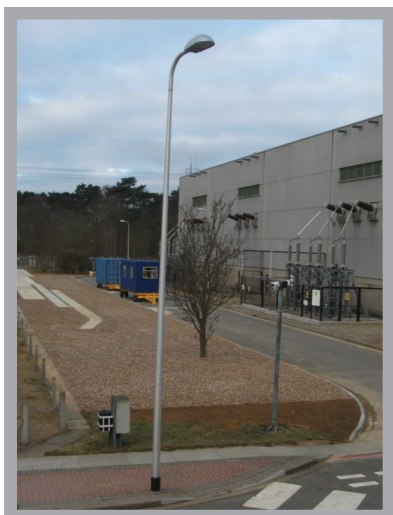
Figure 4: Area restored after excavations
