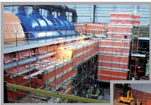
Figure 11: Example of Turbine Hall Asbestos removal
