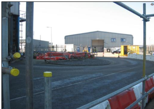
Roads kept clean through implementation of wheel washing
