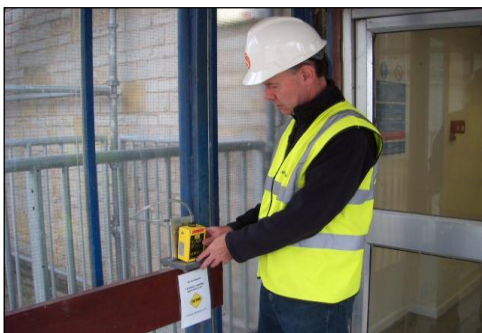
Dust Monitoring In Progress
