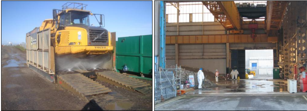
Wheel washing and water spraying to minimise dust generation
