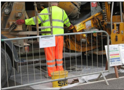
Polythene sheeting to prevent dispersion
