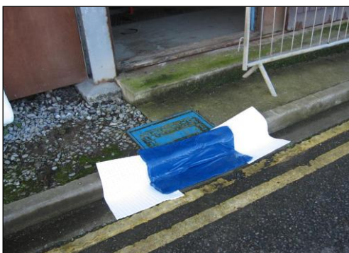
Surface water drain protection
